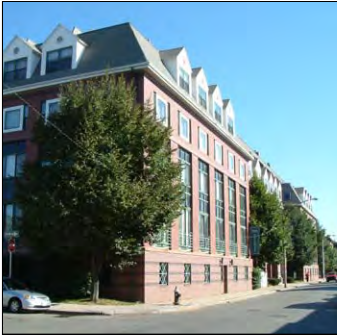
Parking can be integrated into the base of a building above grade while respecting the pedestrian environment. At the Vicomte Condominiums in Allston, the masonry facade at parking level, two story tall windows, and top floor roof and dormers allow a five story building to fit into a small scale residential context. Generous entries are at grade, displacing the parking in critical places.
