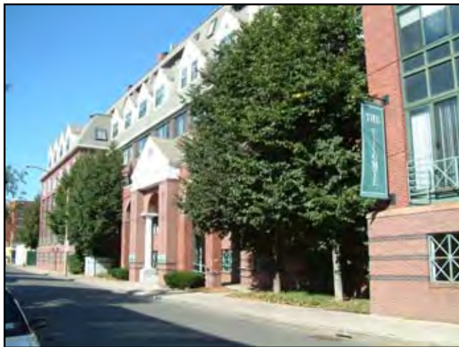
Parking can be integrated into the base of a building above grade while respecting the pedestrian environment. At the Vicomte Condominiums in Allston, the masonry facade at parking level, two story tall windows, and top floor roof and dormers allow a five story building to fit into a small scale residential context. Generous entries are at grade, displacing the parking in critical places.
