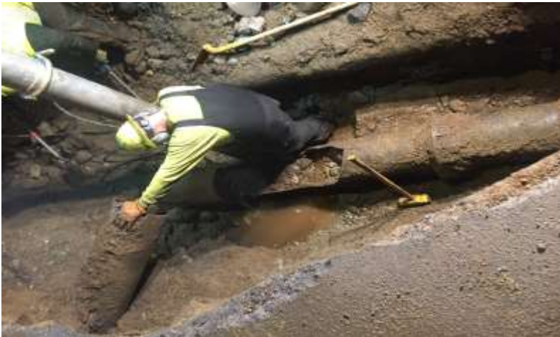
Water Main Break Repair
