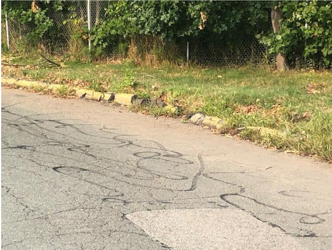
Parkway curb and pavement condition at 200Q
