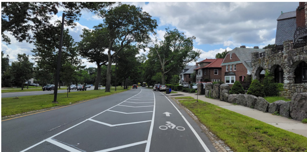
Figure 17: Example of a one-way bike lane
