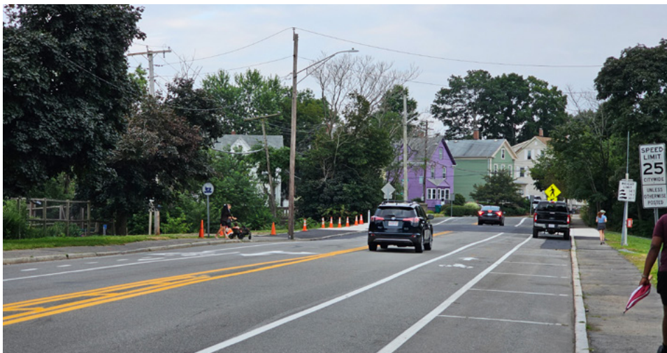
Figure 15: Example of a one-way bike lane
