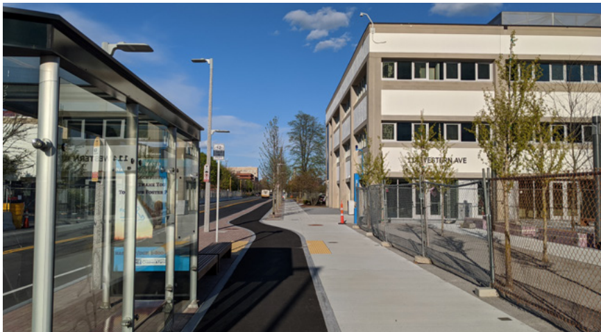
Figure 10: Example of a cross section with protected bike lanes with a curb separation
