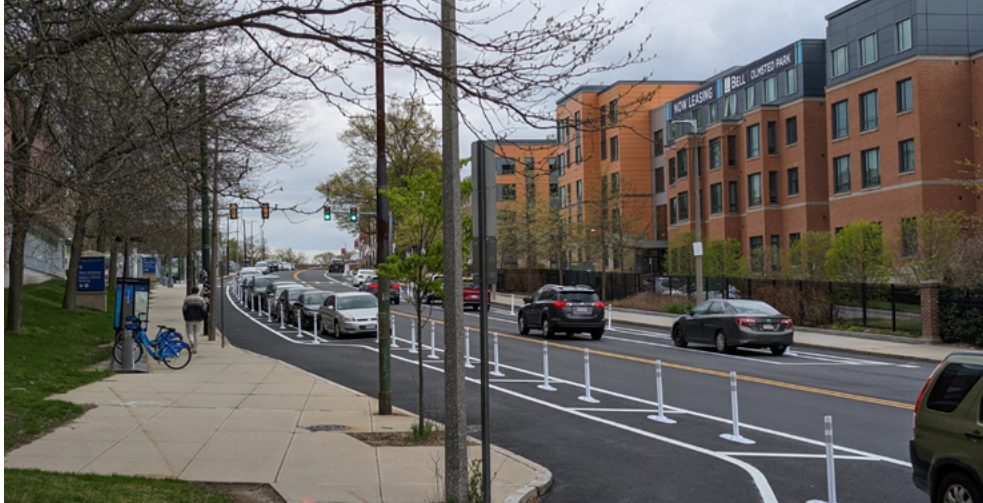
Figure 11: Example of protected bike lanes with parking separation
