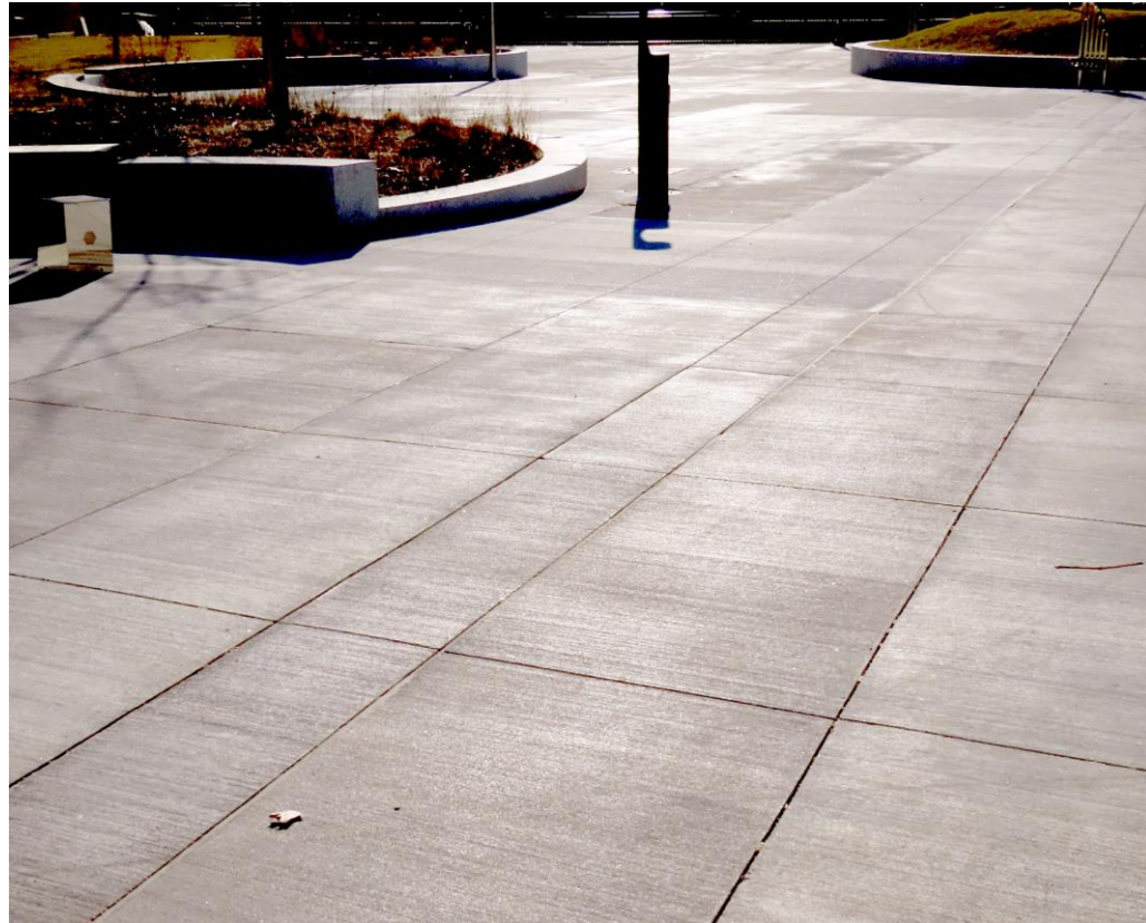
Concrete with Sawcut Joints
