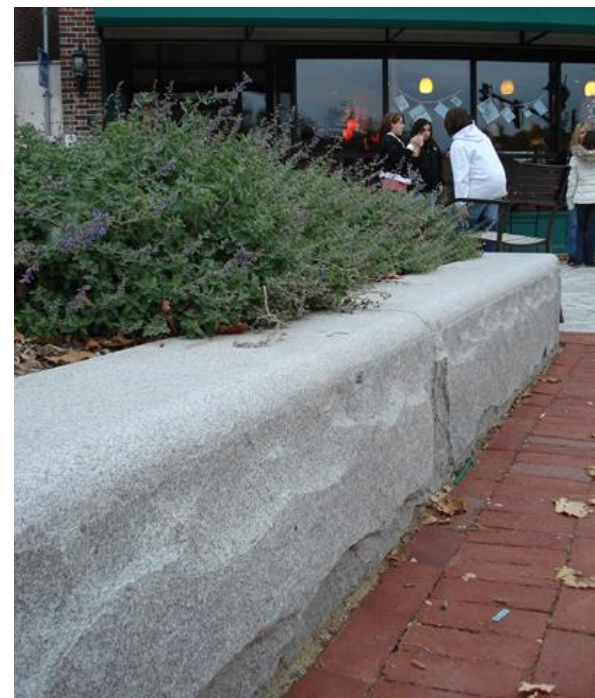
Granite Planter Seatwalls
