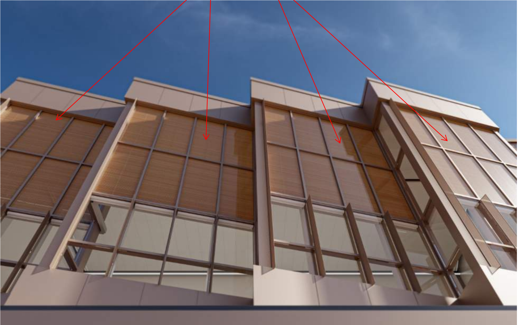
VIEW OF MEDIA CENTER CURTAINWALL AND OKAWOOD IGU
