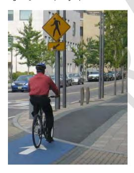
Figure 10: Example of a cross section with protected bike lanes with a curb separation
