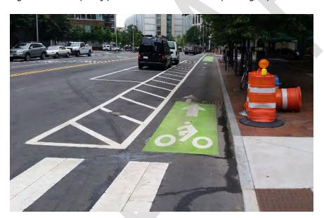
Figure 12: Example cross section of protected bike lanes with parking separation
