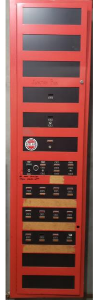
Original zoned fire alarm panel. New addressable panel connects original zones.
