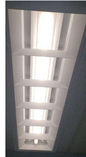
Linear fluorescent lighting retrofitted with T8/electronic ballasts
