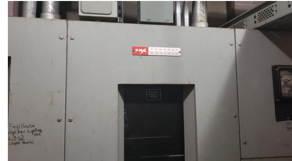
Original Federal Pacific Main Switchboard
