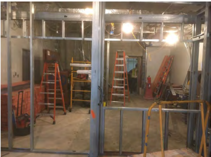
Transaction window, door, and soffit framed in dispatch room
