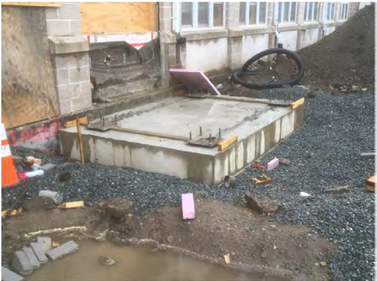
Concrete forms removed from vestibule slab
