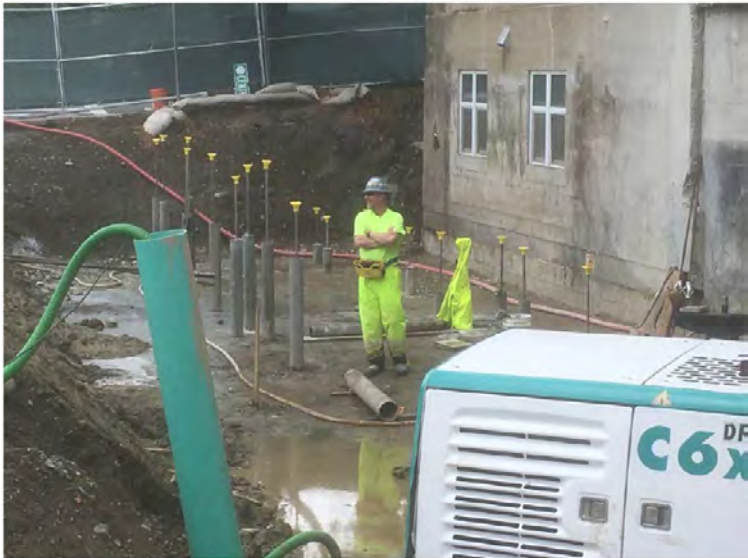
Micro-piles with yellow rebar caps
