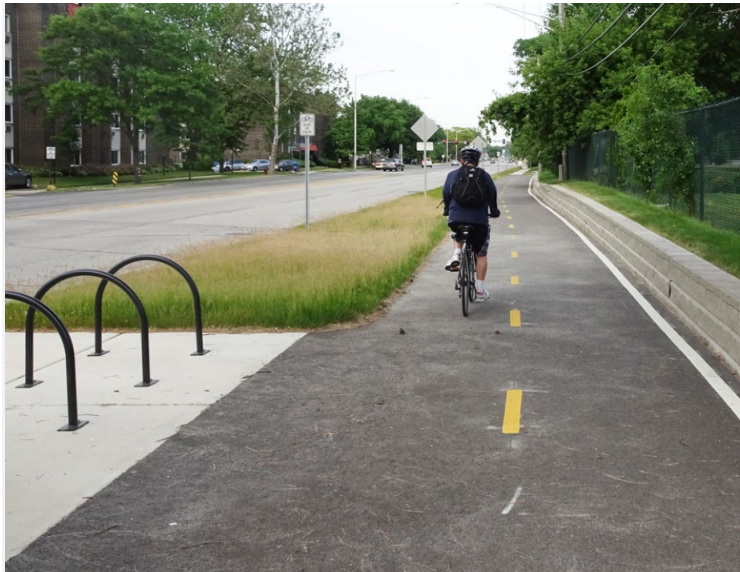
Figure 8: Example cross section of shared use path adjacent to the roadway
