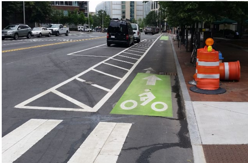
Figure 11: Example of protected bike lanes with parking separation
