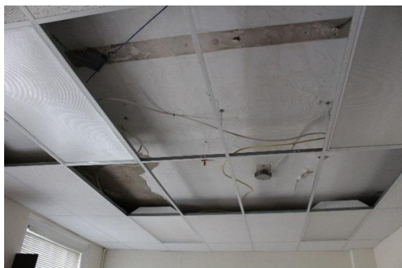
Figure 25: Exposed ceiling wires on second level
