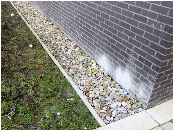
GRAVEL MAINTENANCE STRIP AT BUILDING
