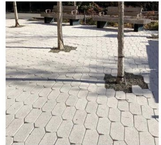
Permeable Unit Pavers at Plaza
