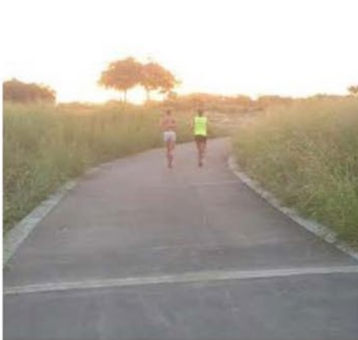
Porous Asphalt Community Path
