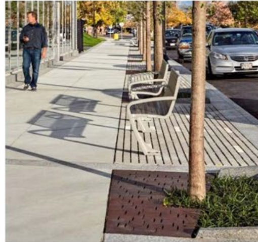
Permeable Paver Furnishing Strip
