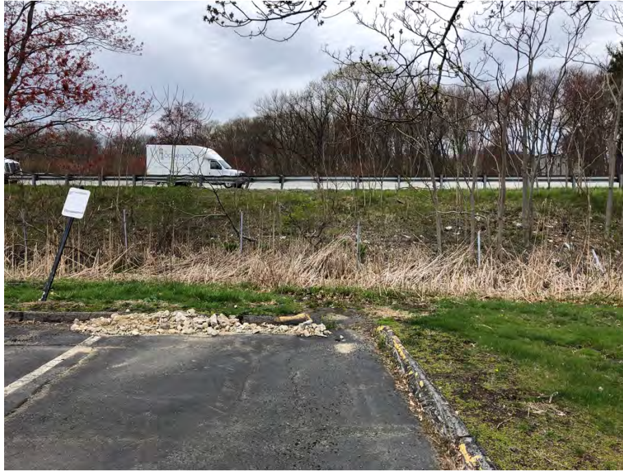
Photo 10: A view of the western stretch of parking lot off of Quannapowitt Parkway. Untreated stormwater runoff from the parking lots and roadway discharge into a narrow upland buffer zone before flowing into the BVW in the center of the photo. The intermittent stream Bank is located within this BVW. The stormwater runoff has eroded the uplands buffer zone and is causing sedimentation of the wetlands. The same situation is occurring off to the left of the photo at the opposite corner of the parking area.
