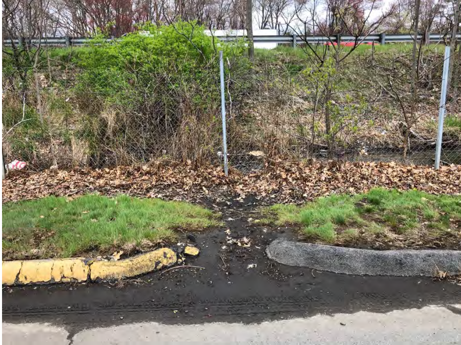
Photo 12: A view of the western stretch of Quannapowitt Parkway. Untreated stormwater runoff from the roadway and parking lots discharge into a narrow upland buffer zone before flowing into the BVW in the center of the photo. The intermittent stream Bank is located within this BVW and can be seen in the center-left portion of the photo. The stormwater runoff has eroded the uplands buffer zone and is causing sedimentation of the wetlands.
