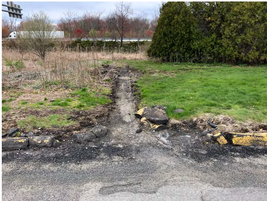
Photo 9: A view of the western stretch of Quannapowitt Parkway. Untreated stormwater runoff from the parking lots and roadway discharge into an upland buffer zone before flowing into the BVW in the background of the photo. The stormwater runoff has eroded the uplands buffer zone and is causing sedimentation of the wetlands. The intermittent stream Bank is located within this BVW. This area appears to have been dug out to improve drainage of the roadway.
