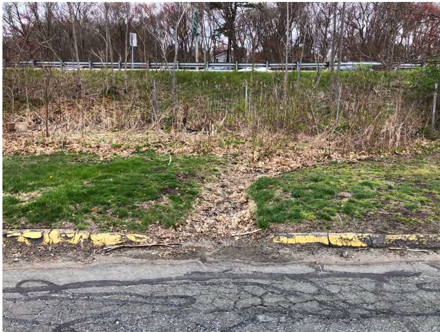
Photo 11: A view of the western stretch of Quannapowitt Parkway. Untreated stormwater runoff from the roadway discharge into a narrow upland buffer zone before flowing into the BVW in the center of the photo. The intermittent stream Bank is located within this BVW.
