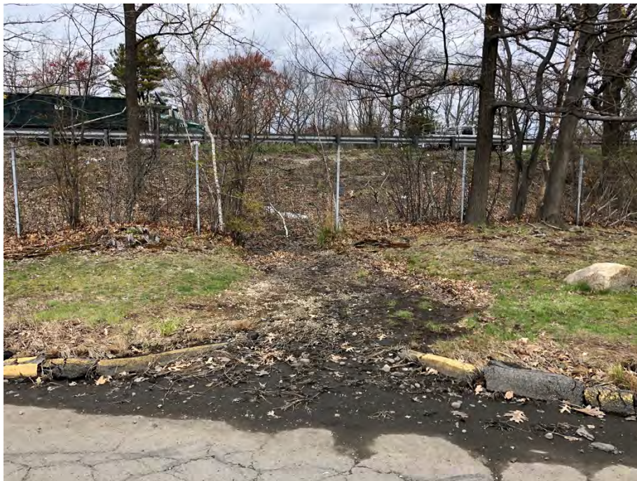
Photo 13: A view of the northern corner of Quannapowitt Parkway. Untreated stormwater runoff from the roadway and parking lots discharge into upland buffer zone before flowing into the wetlands in the center of the photo. The stormwater runoff has eroded the uplands buffer zone and is causing sedimentation of the wetlands.
