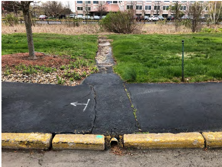
Photo 6: A view from the southern stretch of Quannapowitt Parkway looking toward the perennial stream and BVW. A small pipe inlet can be seen between the yellow curbs. This pipe collects stormwater runoff and directs water and sediment down a paved swale towards the BVW and perennial stream. Sediment can clearly be seen within the swale.
