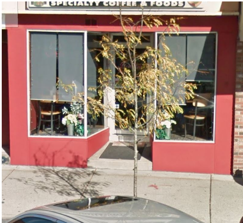
Figure 2: An example of a potential variance needed because the existing floor elevation is higher than the sidewalk and not enough room to construct a ramp.
